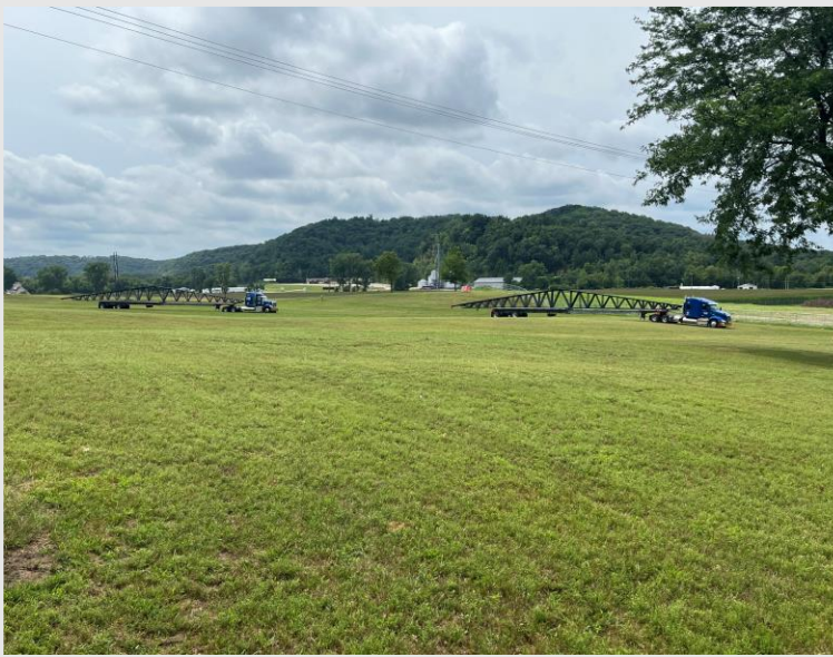
105' Trusses being delivered to the jobsite
