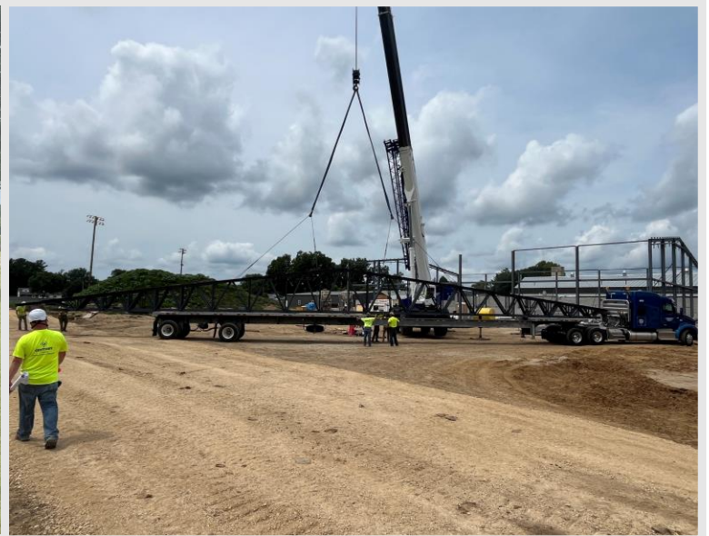
Rigging the Trusses getting them ready to unload
