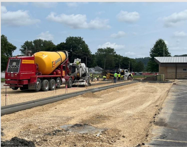
Crews Pouring Curb in the North Parking Lot
