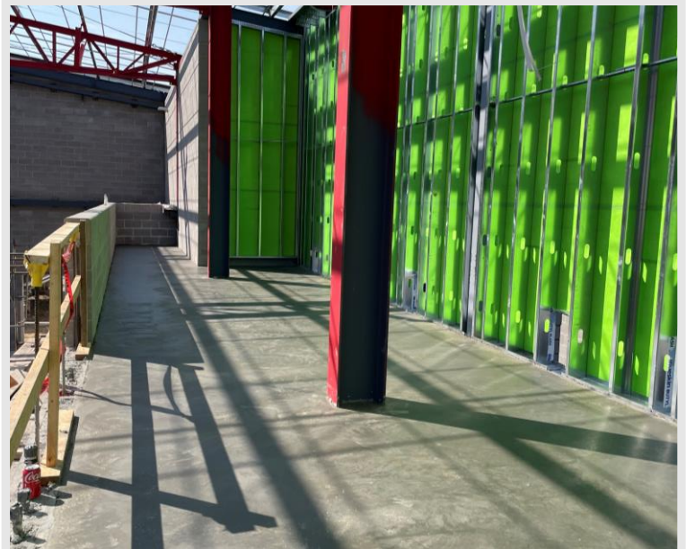
Media Mezzanine Deck had concrete floor poured.
