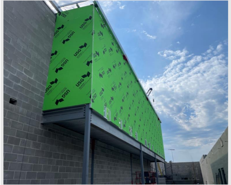
Media Mezzanine is framed and sheathed above new locker room area.
