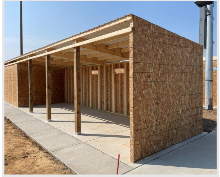
Framing of 4 new Dugouts has begun at the Baseball and Softball.
