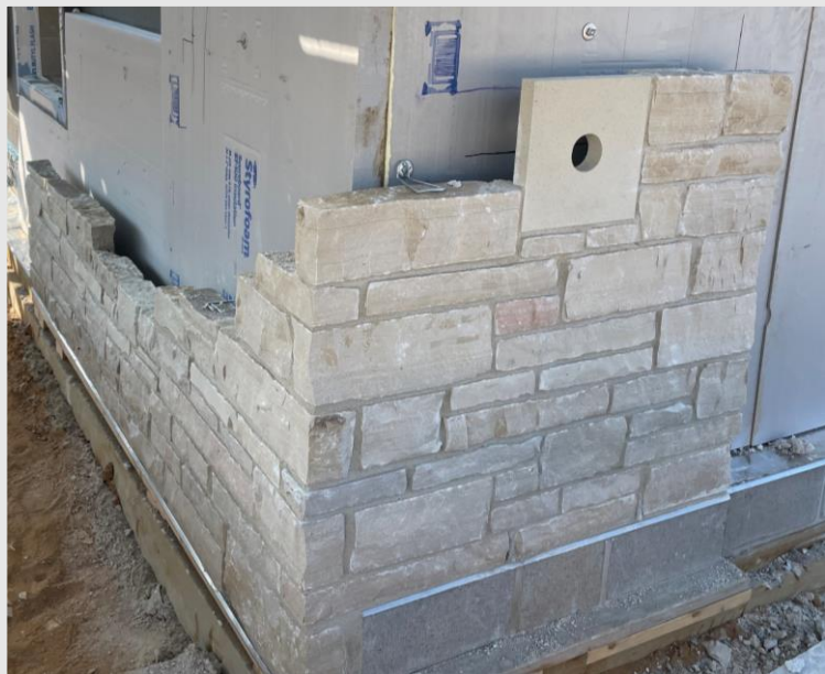
Masons have started stone accent walls near new Admin Offices.
