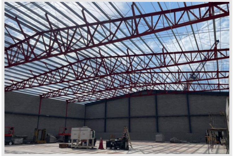
Gymnasium is ready for roofing to begin.
