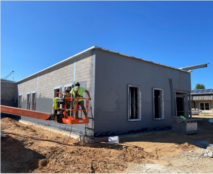
Air & Vapor Barrier is being applied to exterior block walls.
