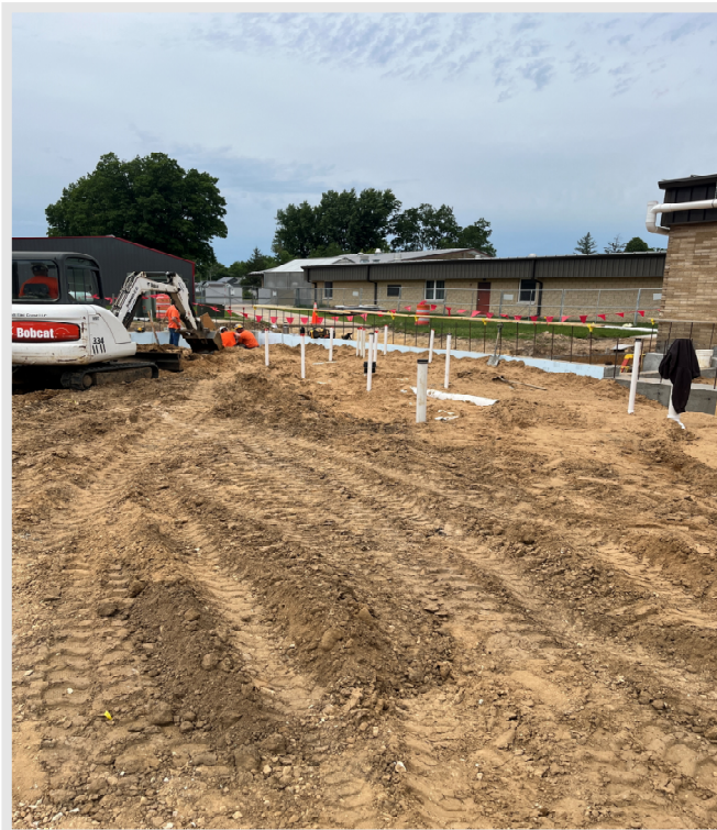
New Plumbing Being Installed in the new Locker Rooms
