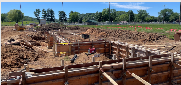
Form Work Set Up for One of the Big Wall Pours
