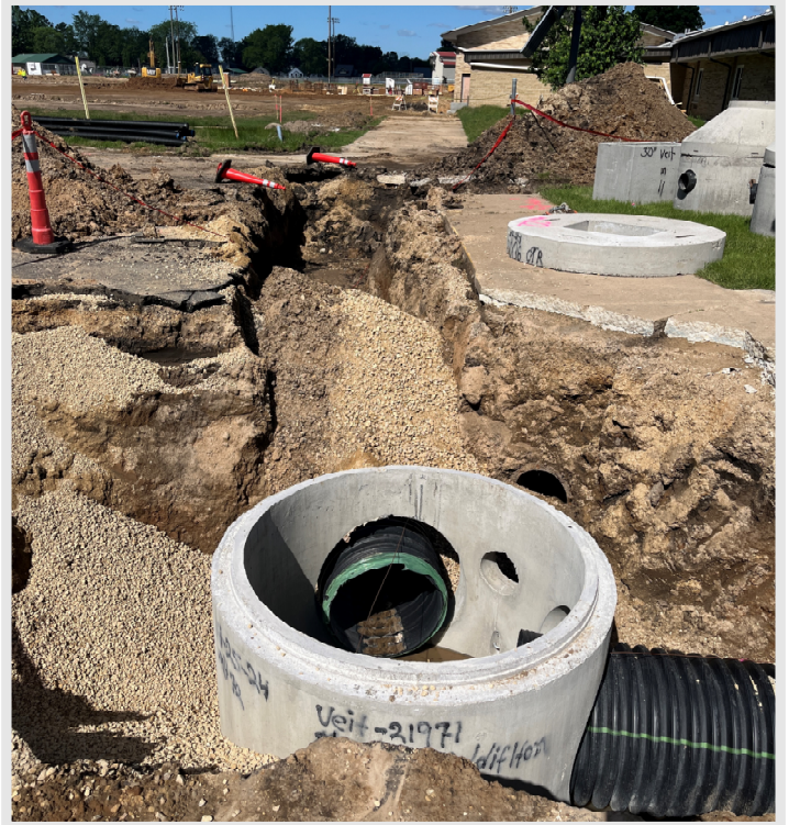
New Manhole and Storm Piping in the East Parking Lot
