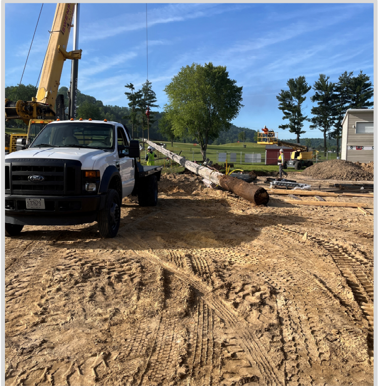
Schmidt Electric Taking Down an Existing Light Pole
