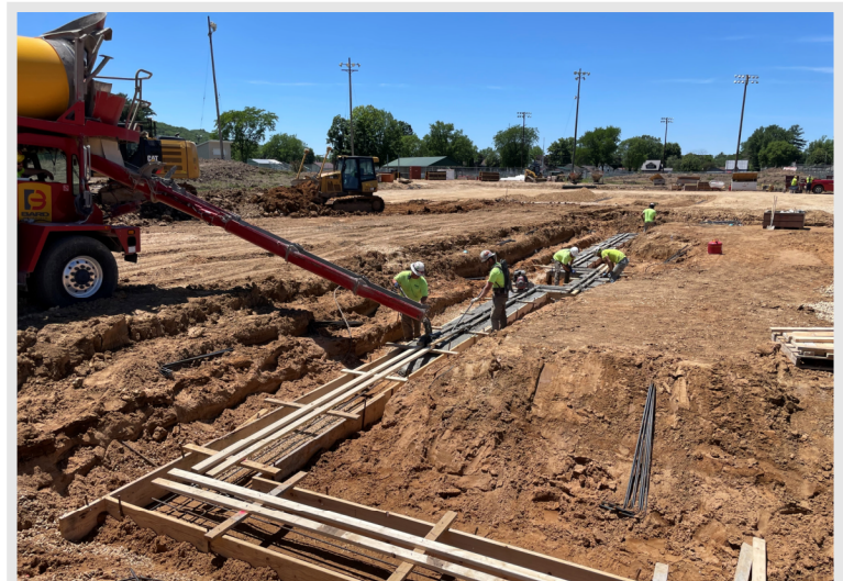
Crews Working Hard to Get a Long Stretch of Footing Poured
