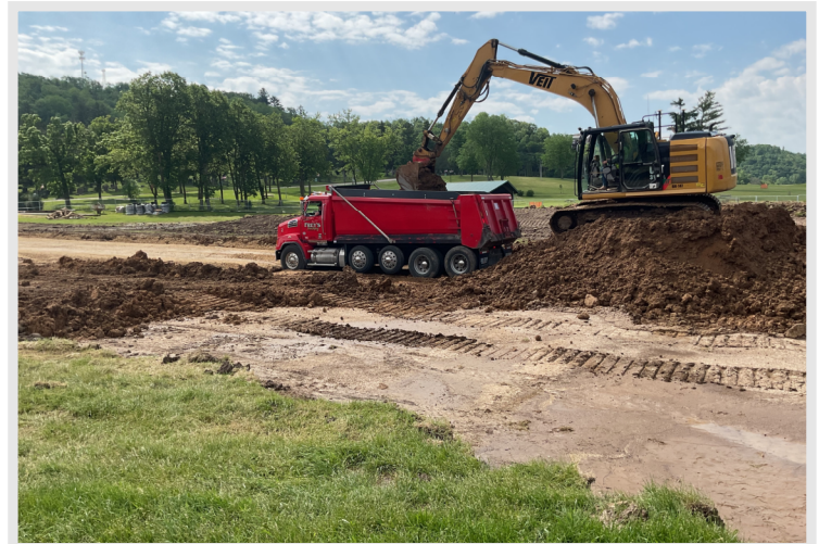
Local Trucking Company - Frey Trucking hauling material
